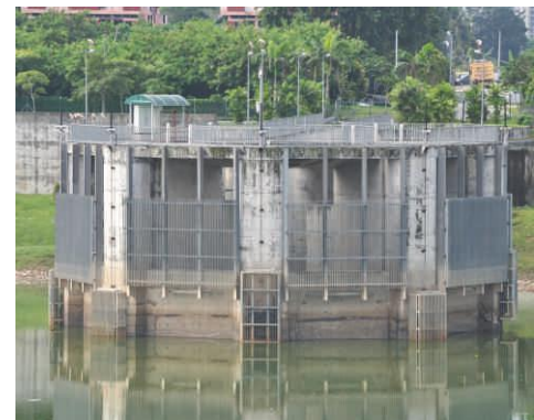
Sluice Gate & Trash Screen at Kerajaan Storm Water Management and Road Tunnel Project, Kuala Lumpur, Malaysia
