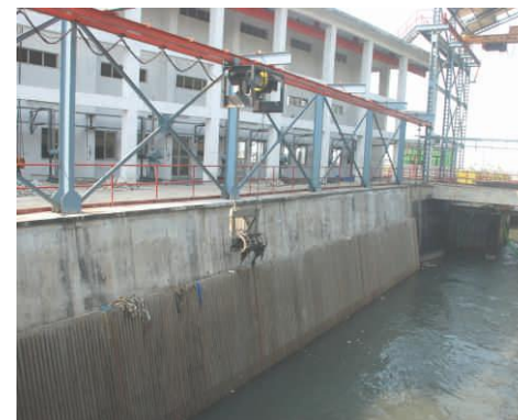
Suspended Trash Rake Screen and Sluice Gate at Haji Ali Storm Water Pumping Station, Mumbai, India
